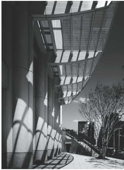
Detail of Mori Tower canopy
