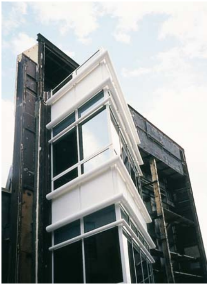
Curtain wall performance mock-up
