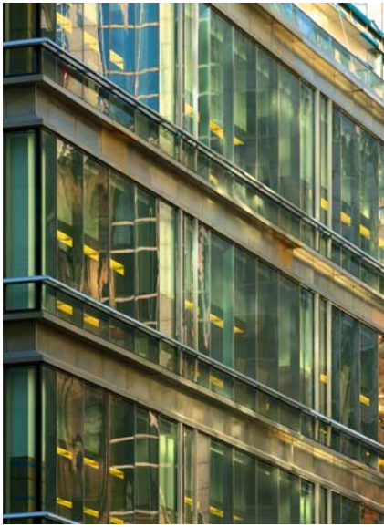
Detail view of lower office level curtain wall
