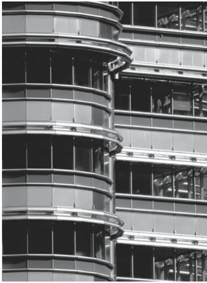
Detail of Petronas Towers curtain wall
