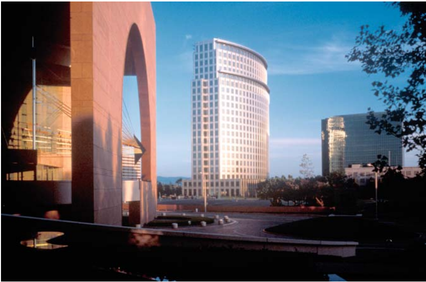
View of north-west elevation
