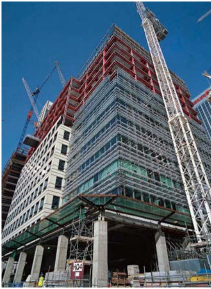
Curtain wall installation
