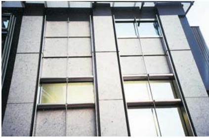
Curtain wall visual and performance mock-up
