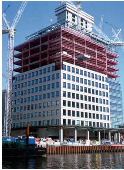
Curtain wall installation
