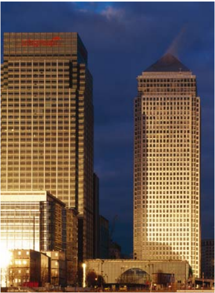
East view of One Canada Square from Canary Wharf
