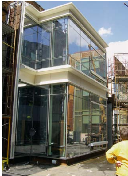
Tower curtain wall mock-up
