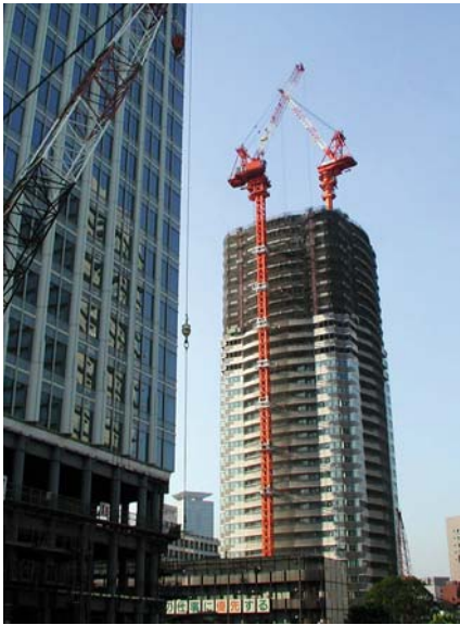
South elevation under construction
