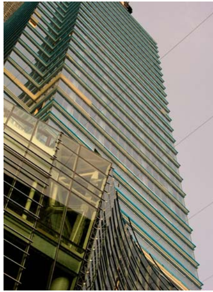
View of east elevation from Beacon Court
