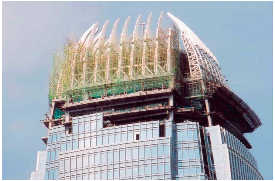
Tower top under construction
