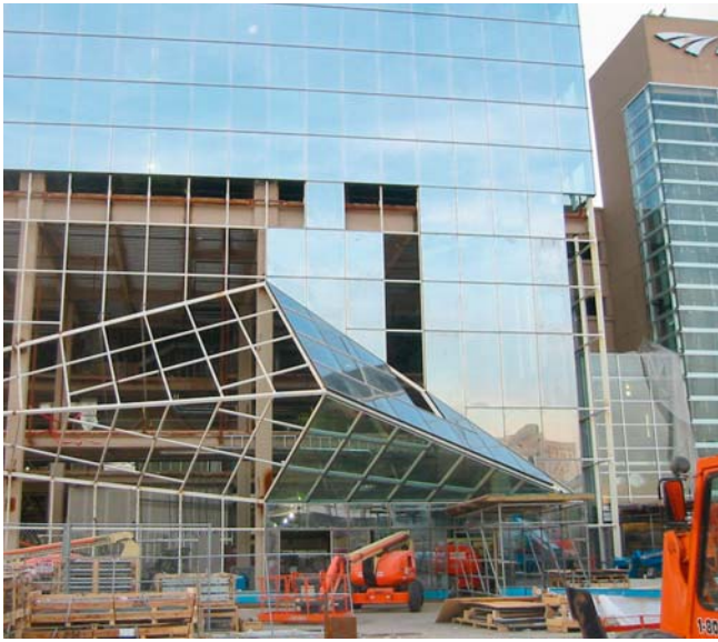
Canopy under construction East elevation under construction
