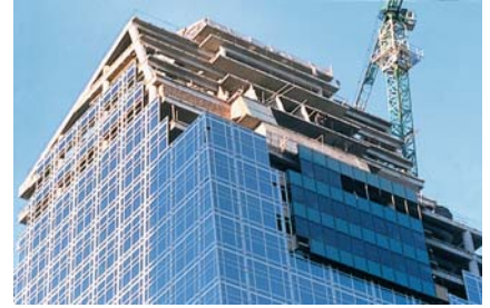
Tower top under construction
