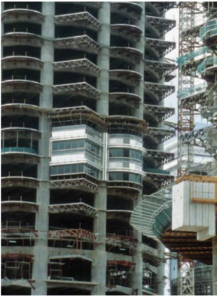
Tower base under construction
