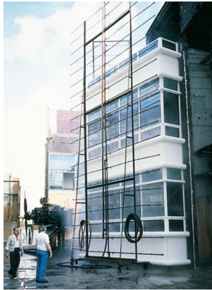
Curtain wall performance mock-up
