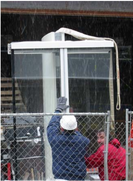
Overture Hall lobby curtain wall visual mock-up
