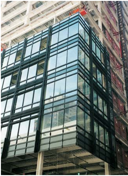
Curtain wall under construction
