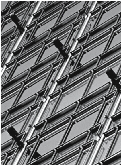
Detail of Cheung Kong Center curtain wall
