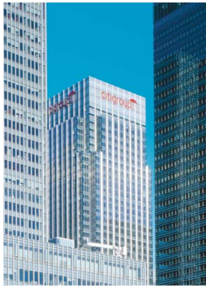
View of tower setbacks
