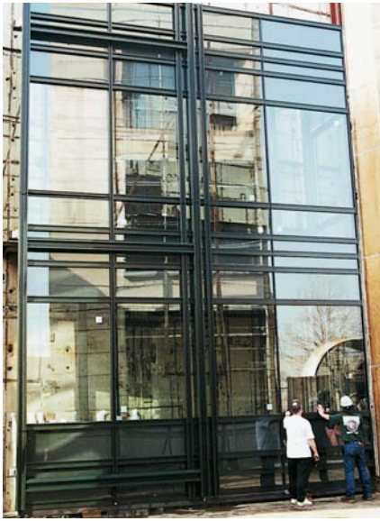
Curtain wall performance mock-up
