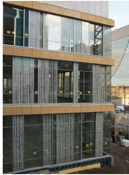
Typical fritted window wall (birch tree pattern)
