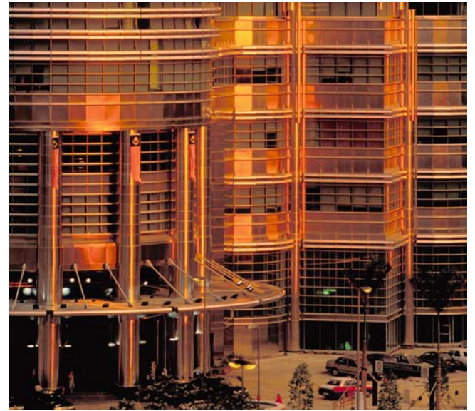
Detail view of tower base at sunset
