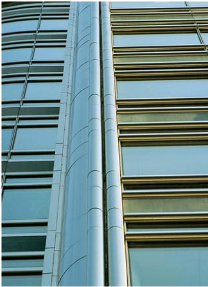
Detail view of stainless steel-sheathed columns
