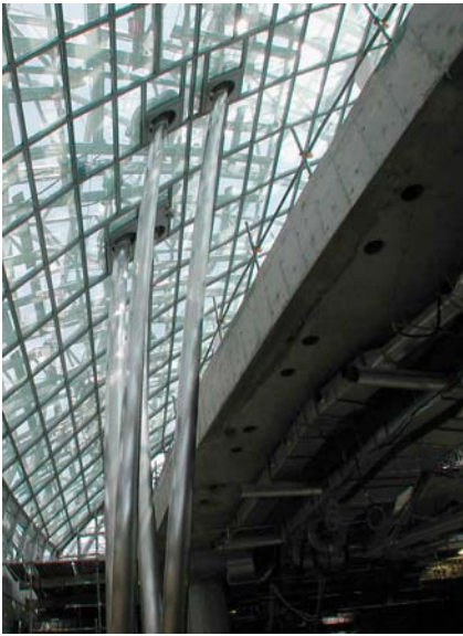
Stainless steel stalk passing through atrium curtain wall
