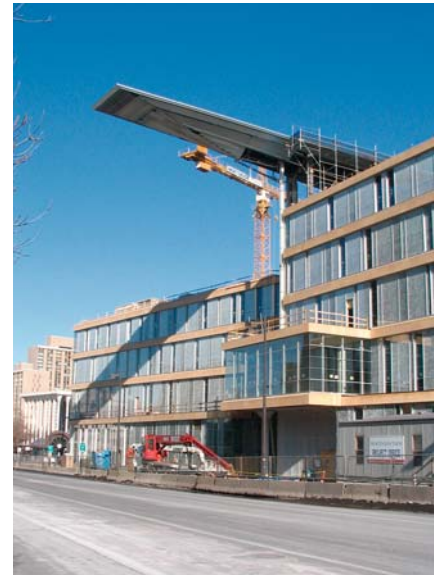
West elevation under construction
