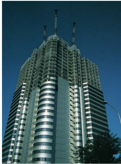
Tower under construction
