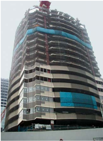
Tower base under construction
