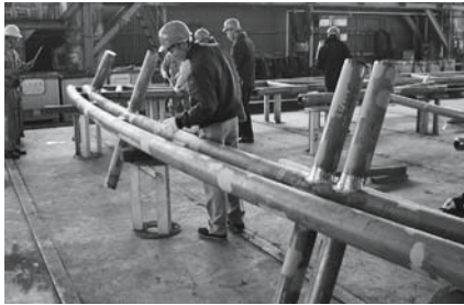
Sculptural form under construction, National Museum of Art, Osaka
