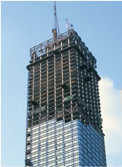
West elevation during curtain wall installation
