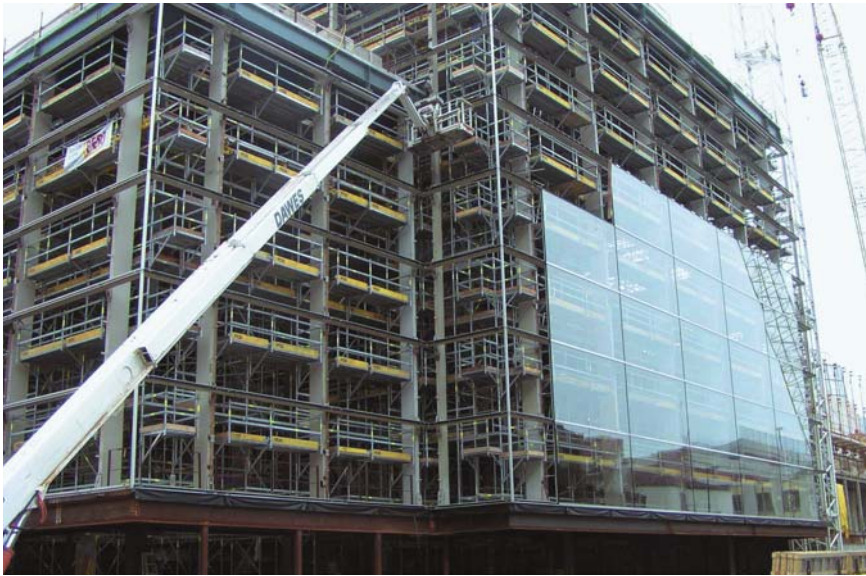
North elevation curtain wall installation
