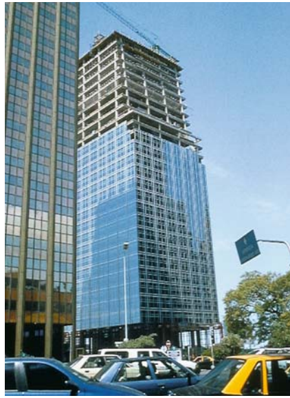
Building under construction from Avenida Alem
