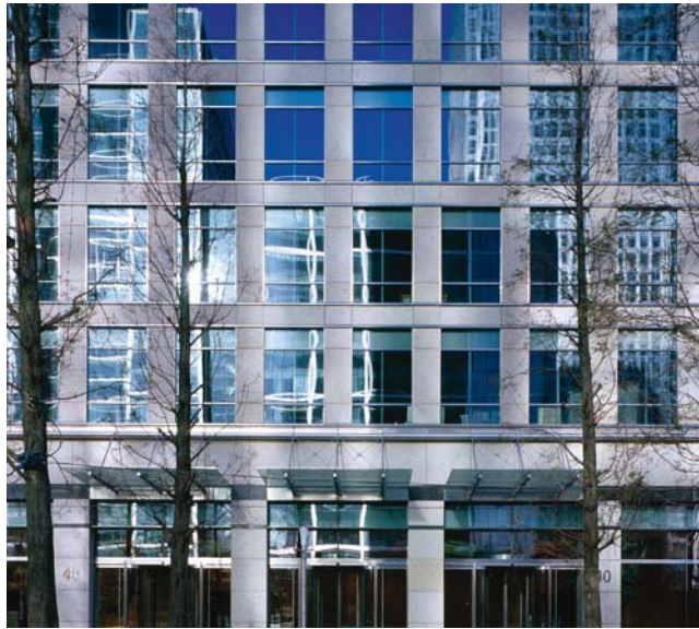
Detail view of curtain wall
