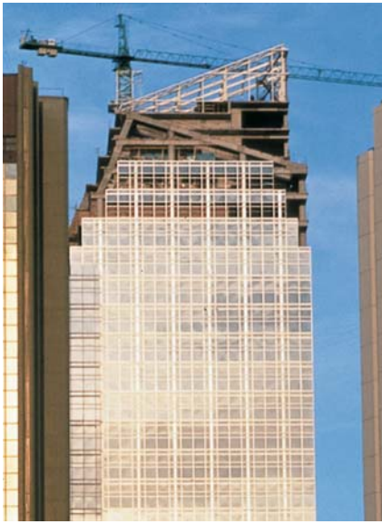
Tower top curtain wall installation
