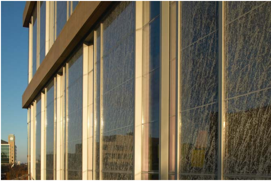
Typical fritted window wall (prairie grass pattern)
