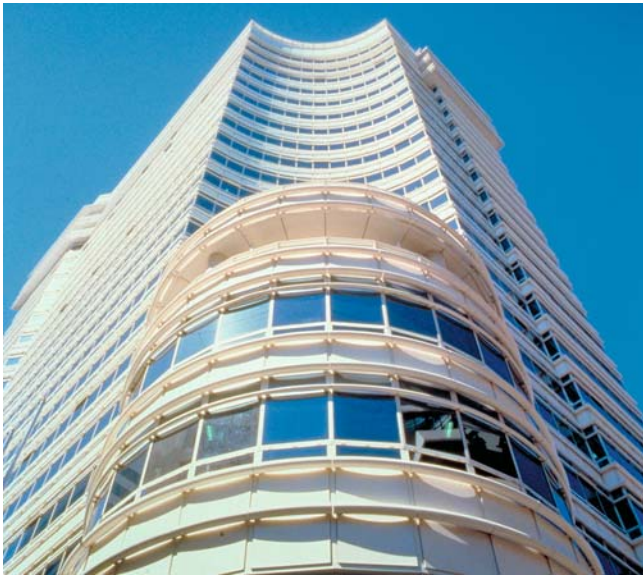
Detail view of corner drum
