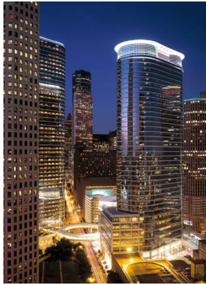
View down Smith Street of west elevation
