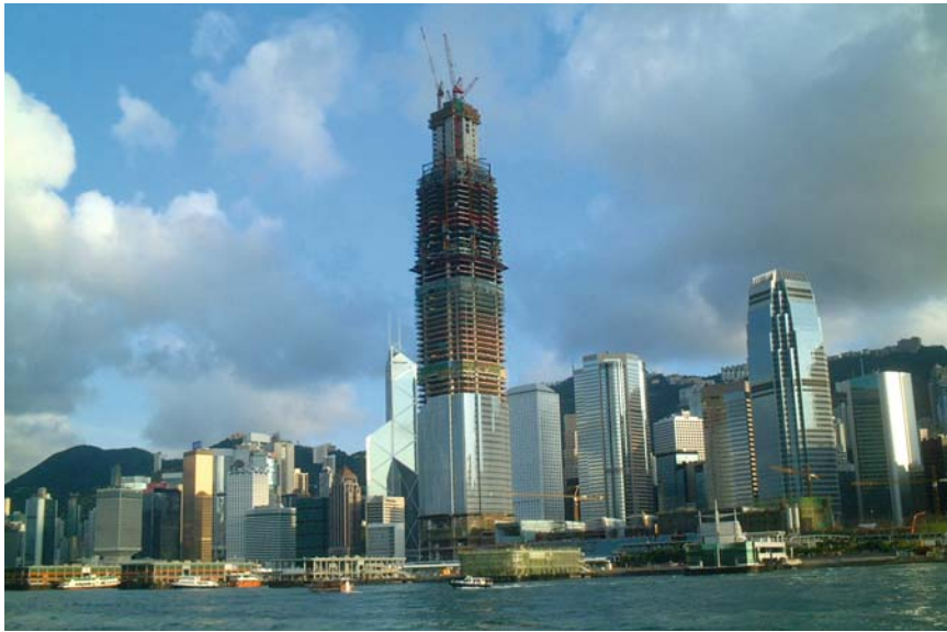
North-west view from Victoria Harbour of construction progress
