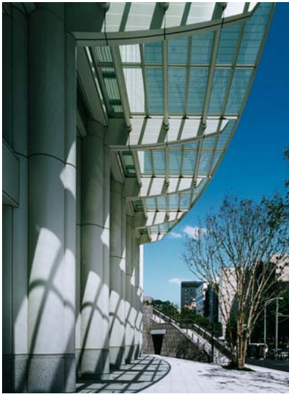
Detail view of canopy
