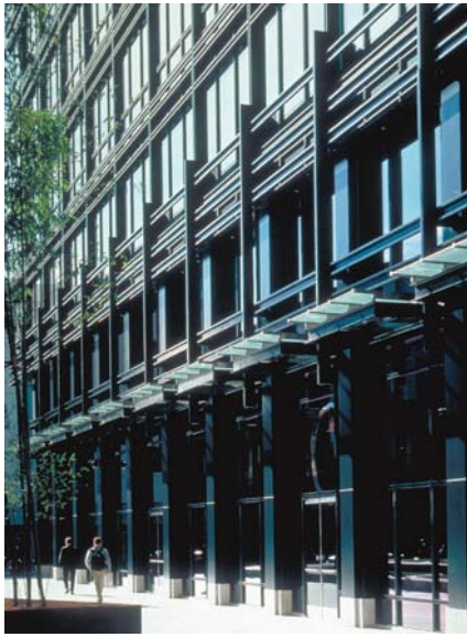
View of plaza level colonnade
