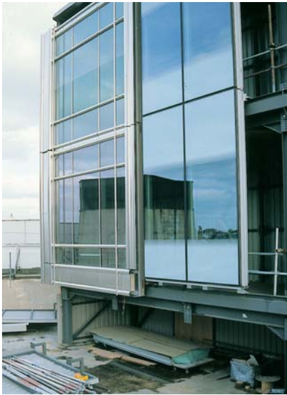
Curtain wall visual and performance mock-up
